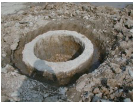
图1 PCC桩 Fig.1 PCC pile
